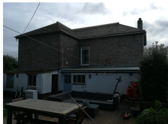
Photo 2. Showing the rear of the house
