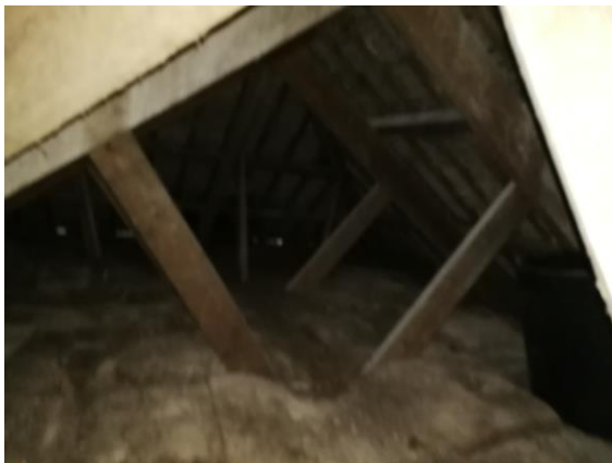
Photo 3. Showing roof void in return arm
