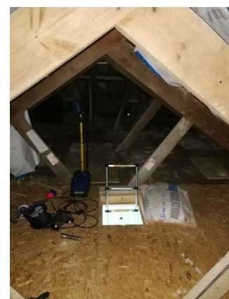
Photo 4. Showing roof void over main part of the house where works have been done
