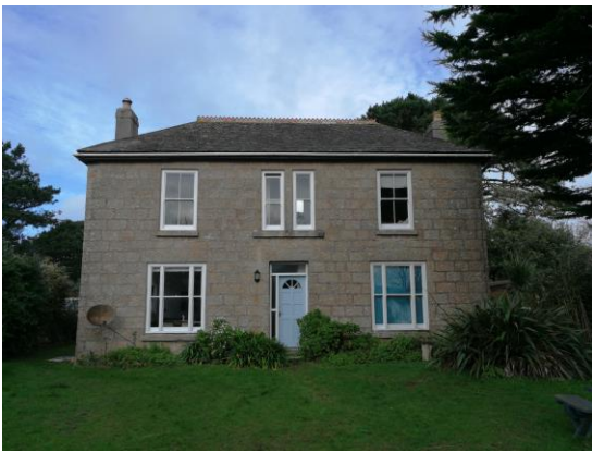
Photo 1. Showing the front of the house
