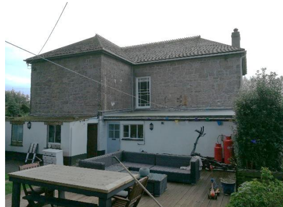
Photo 2. Showing the rear of the house
