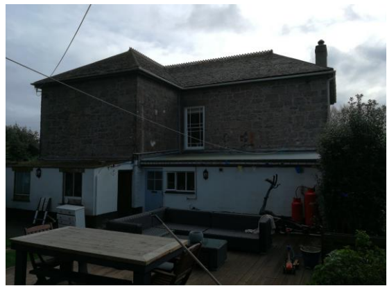
Photo 2. Showing the rear of the house
