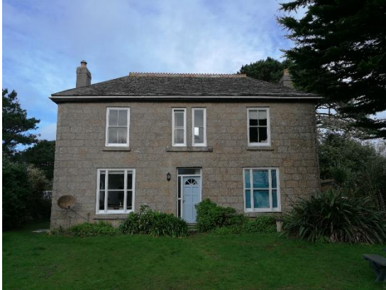
Photo 1. Showing the front of the house
