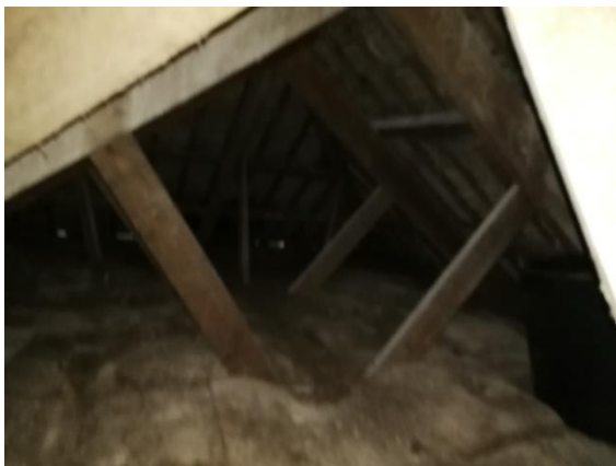
Photo 3. Showing roof void in return arm
