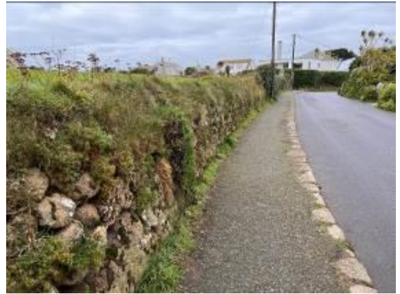
Photo 02 – Showing the eastern boundary where the Cornish Hedge is level with the Circus Field sward to the west (left) but rises above the offsite pavement to the east (right).
