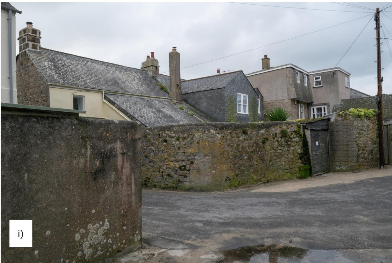
i) Looking southwest at the rear elevations of Parkside, Armorel Cottage and Number 5
