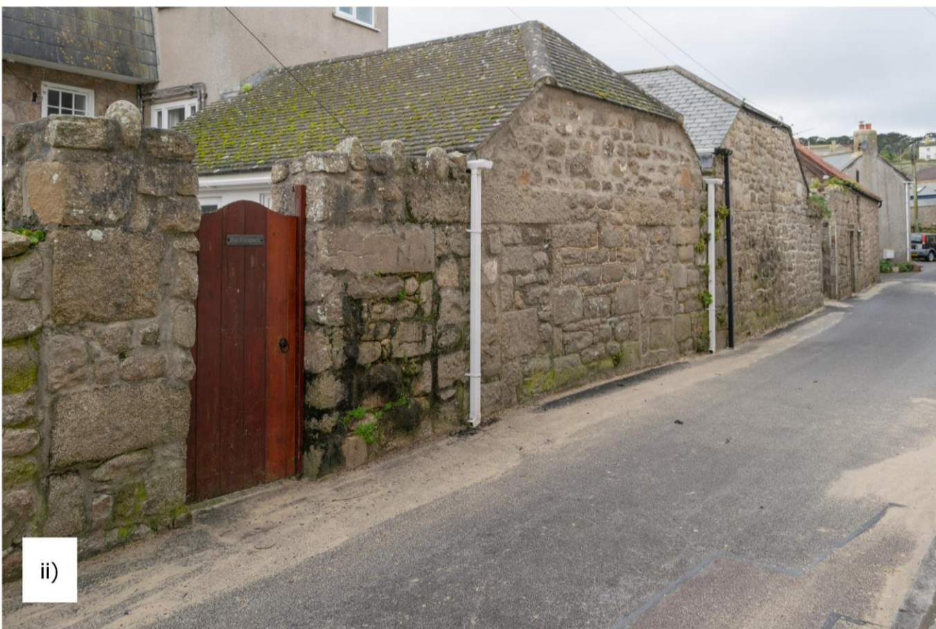
ii) The 19th century sheds to the rear of the three westernmost cottages in the row, likely reflecting the maritime industrial character of Thoroughfare in the 19th century
