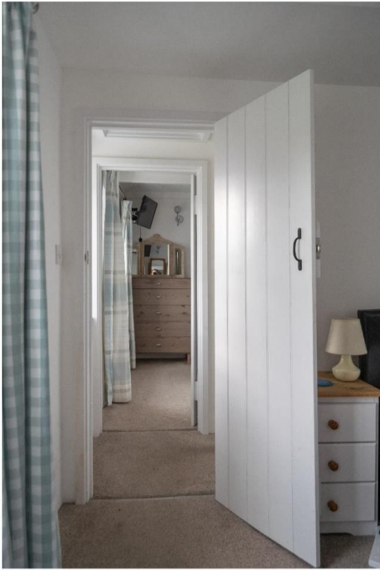
i) modern doorways within plasterboard stud walls of first floor
