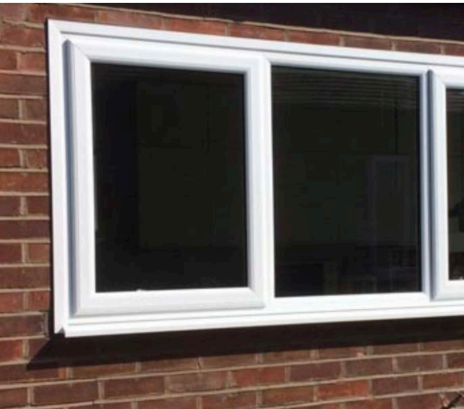
Poorly proportioned uPVC window.
