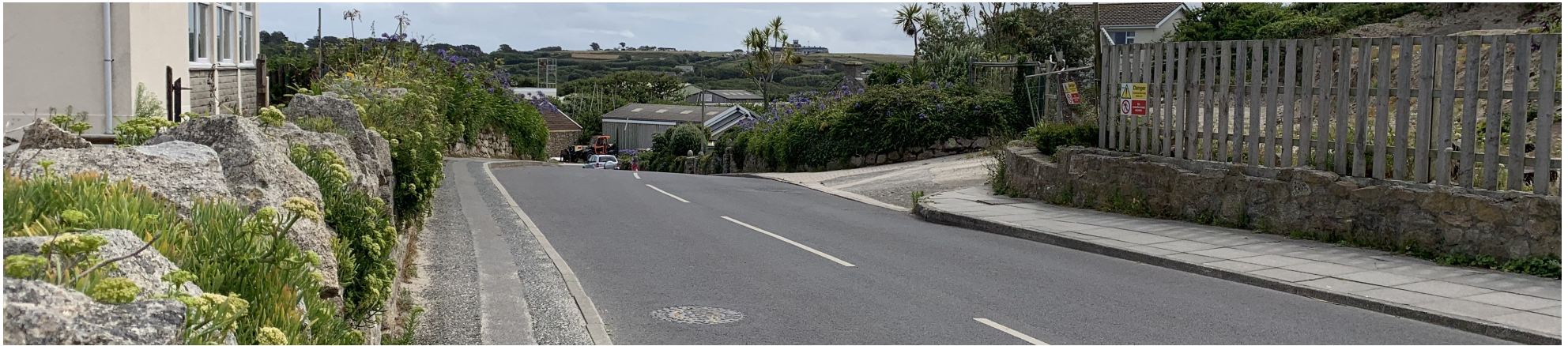
View A from northern footpath on the crest of Telegraph Road looking East opposite the existing site entrance.
