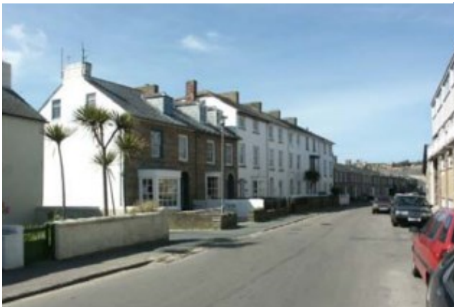
Terraced Housing with defensible front walls along Church Street looking east.
