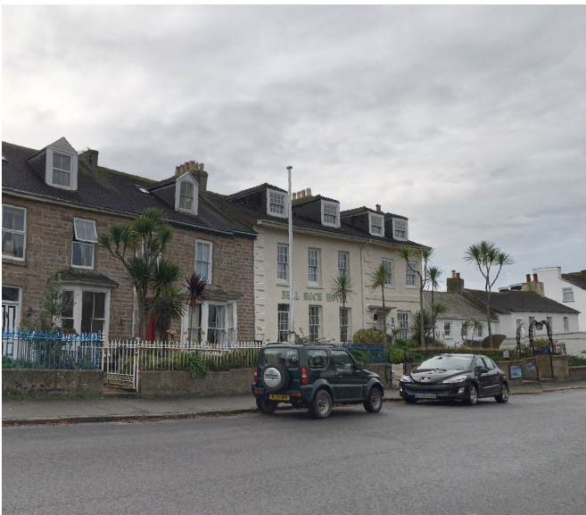
View from Church Street showing 2.5 & 3 storey terraced dwellings
