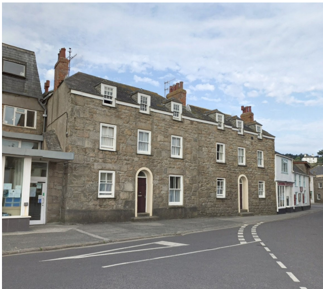
View from the parade showing 2.5 storey buildings with dormers intercepting the eaves
