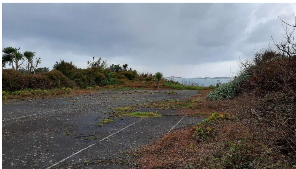
Figure 6: Developed land, sealed surface associated with a former tennis court; view north-west. Scrub and introduced shrub vegetation is encroaching around the edges.
