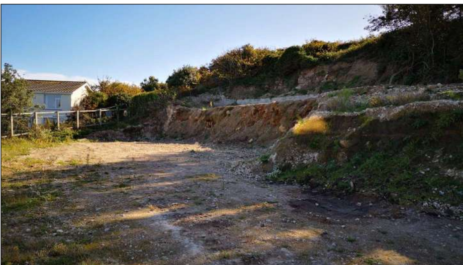
Plate 6: View looking east across the northern part of the application area, showing fragments of stone and concrete retaining walls associated with former school buildings
