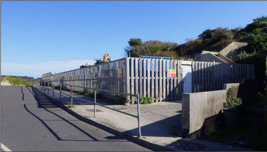
Plate 1: View looking east from Telegraph Road towards the application area rising to the southeast, with extant modern stairwell visible in the slope
