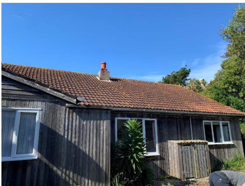
Figure 3: View of the east elevation of Racket Town.
