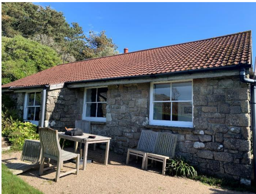
Figure 2: View of the west elevation of Racket Town.
