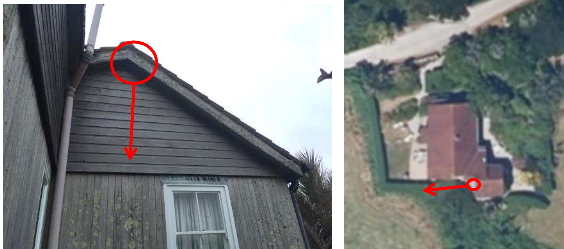
Figure 7: West elevation (left) and aerial view (right) of the south-east projection, showing emergence location of a single common pipistrelle bat on 25 th June 2020.
