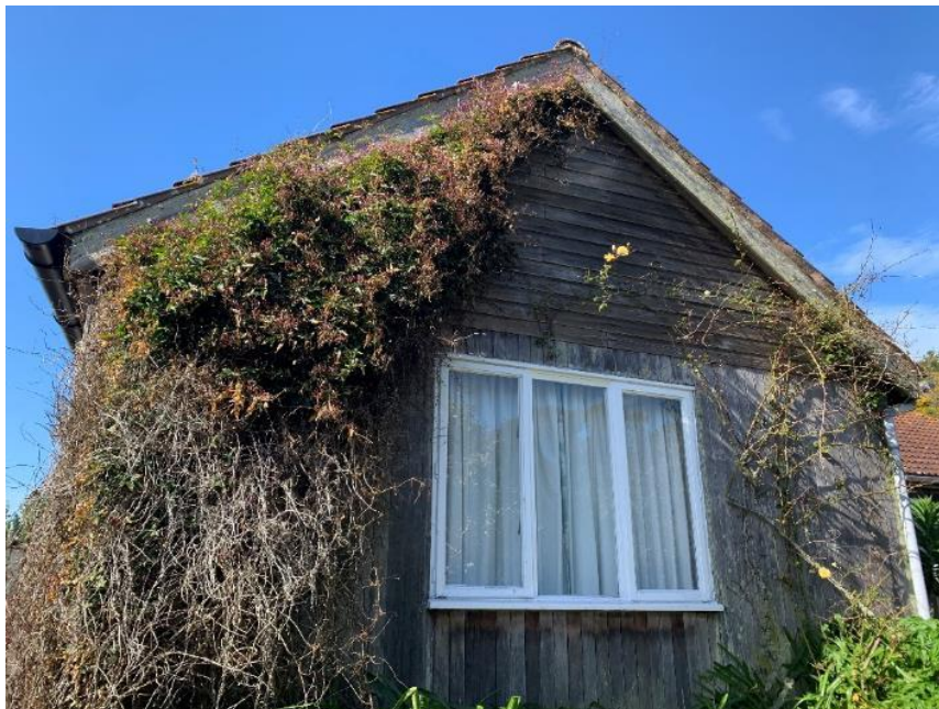
Figure 5: View of the eastern elevation of the south-east projection of Racket Town.
