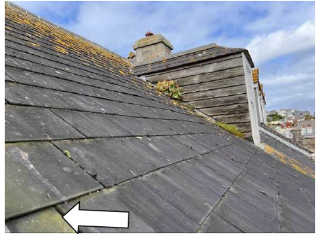
Photograph 2: An example of occasional lifted tiles in B&W A along with the timber-clad dormer.
