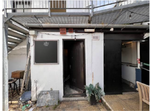
Photograph 14: Showing B&W E on the ground floor
