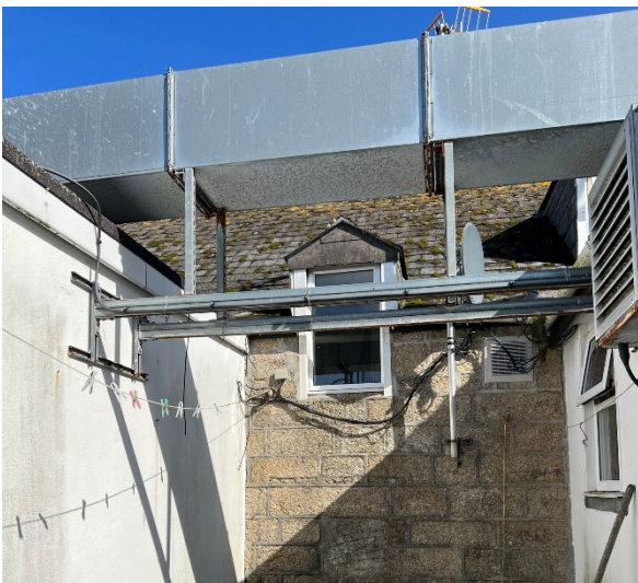
Figures 3-4: Existing extract ductwork
