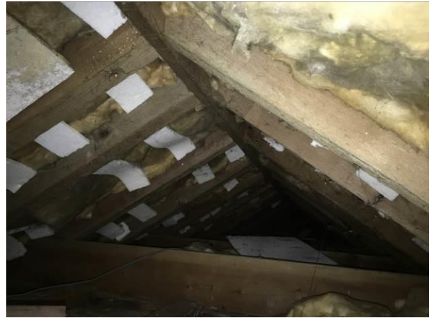
Photograph 8: Showing the main loft above the tie-beam in the main dwelling.
