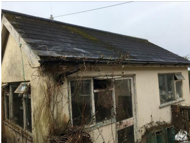
Photograph 9: Showing the single-storey garage.
