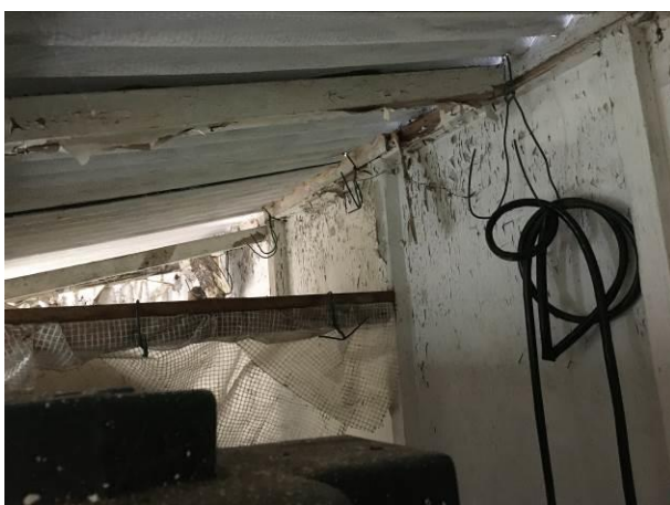
Photograph 11: Showing the roof of the canopy sheltering the oil tank.
