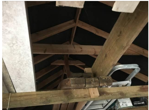
Photograph 10: Showing the interior of the single-storey garage with A-frame timbers and well-fitted underfelting.
