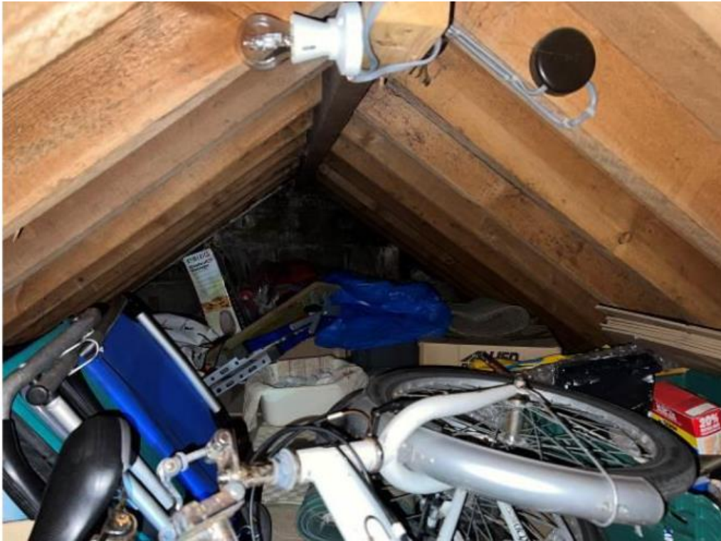
Pl.8: Machine-sawn timbers in the roof space of the rear range.
