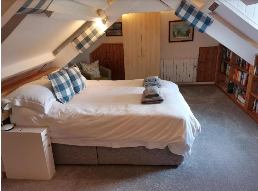
Pl.6: Attic bedroom in the front range, showing truss and purlins.
