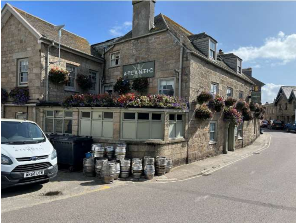
The Atlantic Inn (North & West Elevation)
