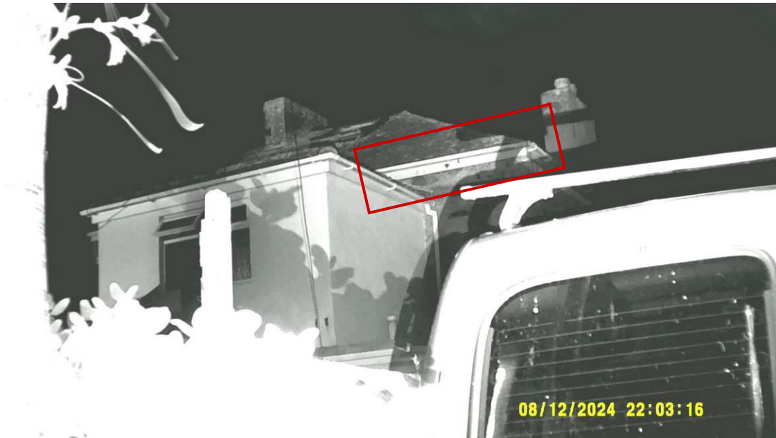
NVA1 – showing a screenshot from the Nightfox Whisker at position NVA1. This is covering the northern side of the eastern aspect. The fascia (potential access feature) is indicated with the red box.
