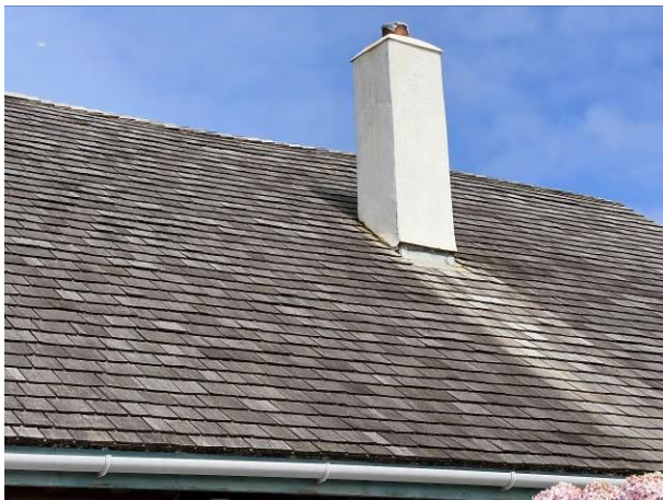
Photograph 3: Showing the chimney set within the shingle roof
