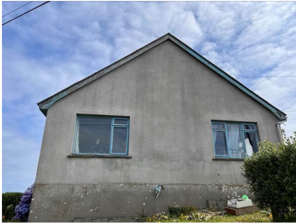
Photograph 1: Showing the southern gable of the property
