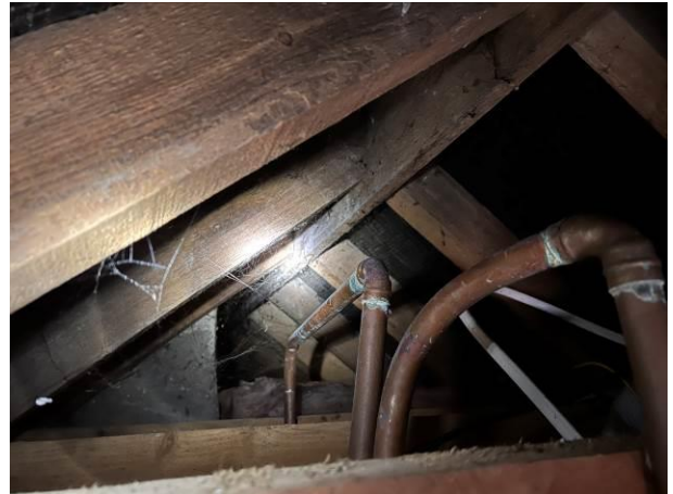
Photograph 2: Showing the small apex void as viewed from the small hatch
