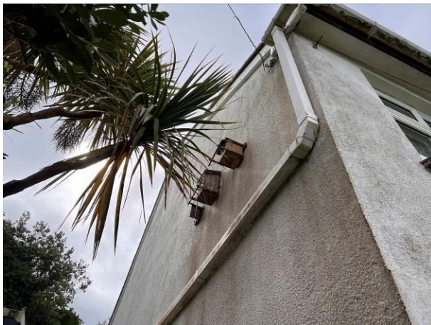
Photograph 9: Showing the bird boxes on the northern gable
