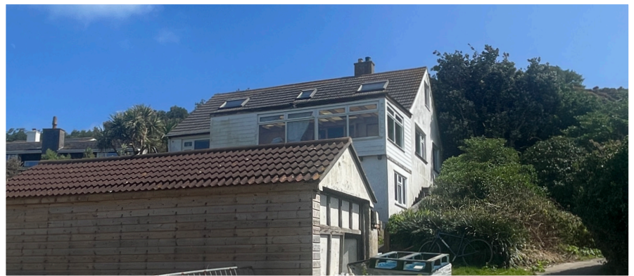
Existing view of the house
