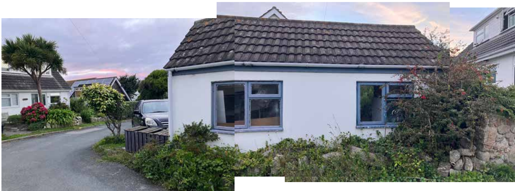
Side elevation to garage, with existing bin storage and parking to the front
