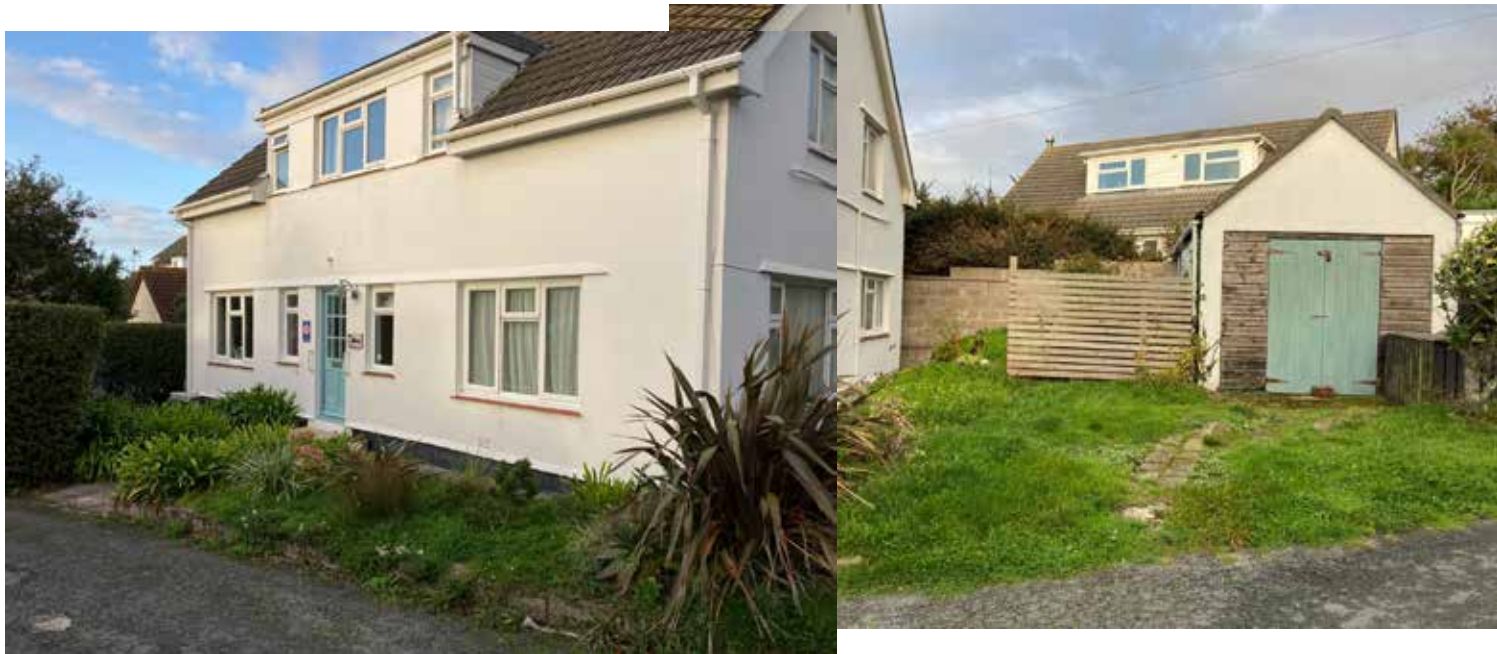
front and side elevation to Nundeeps, showing side raised garden and garage with car parking area
