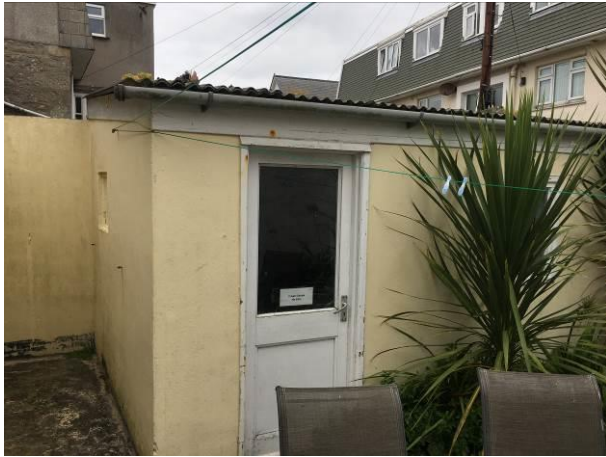
Photograph 7: Showing the Garage in the courtyard garden of the property.
