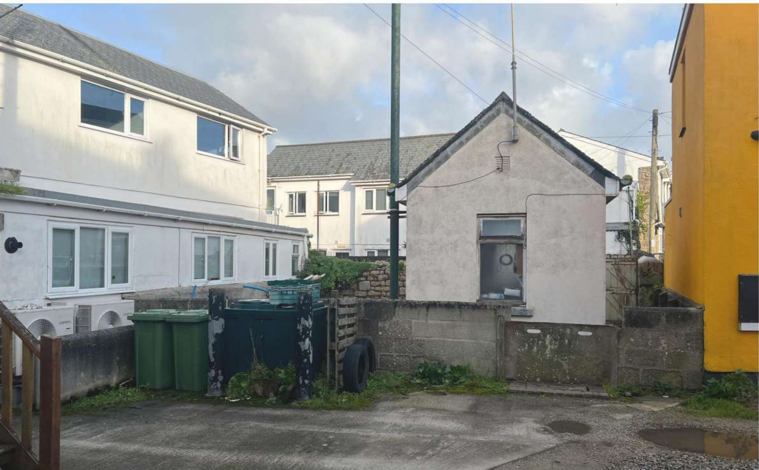
Western Approach; Existing
