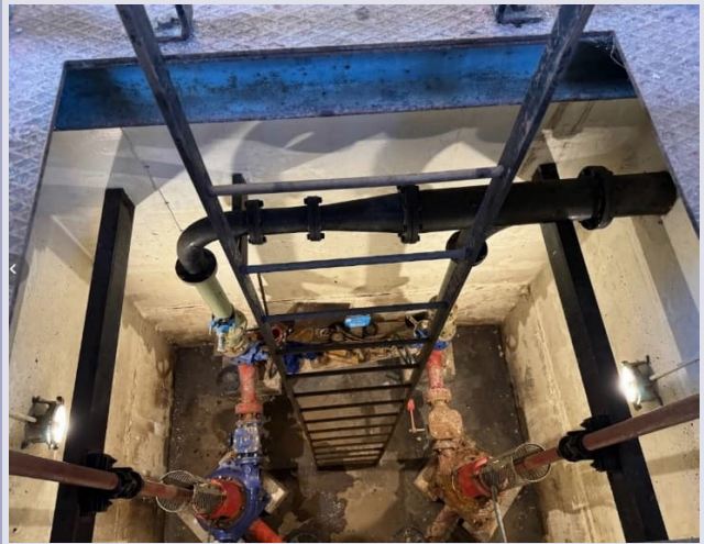
Dry well configuration with access ladder
