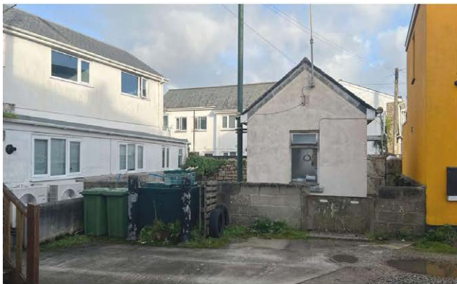
Western Approach; Existing
