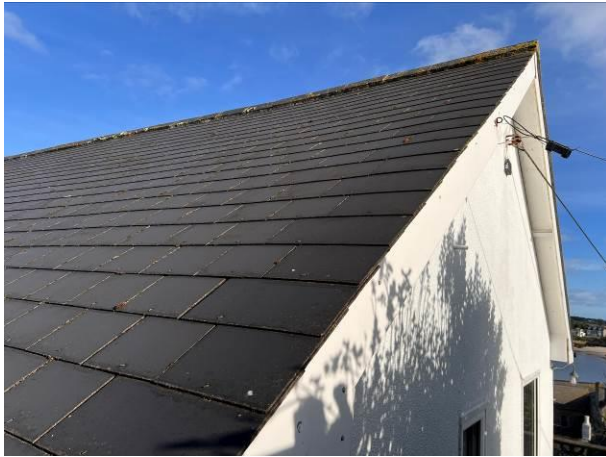
Photograph 1: Showing the well-fitted dry-laid natural slate tiles
