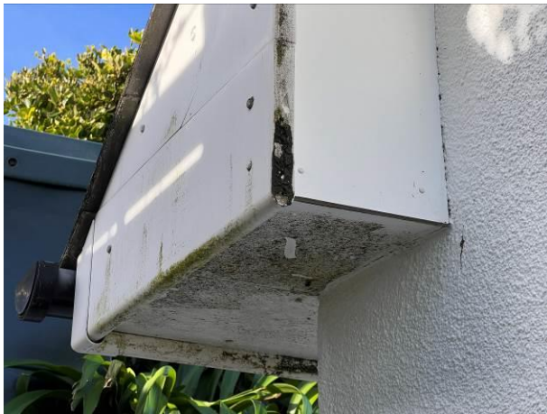
Photograph 3: Showing an example of the well-fitted soffits
