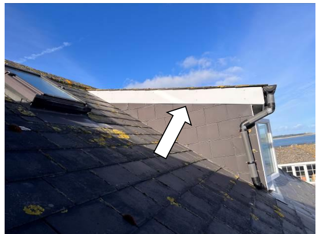
Photograph 6: Showing the side of the dormer – the fascia overtopping the hanging tiles is indicated
