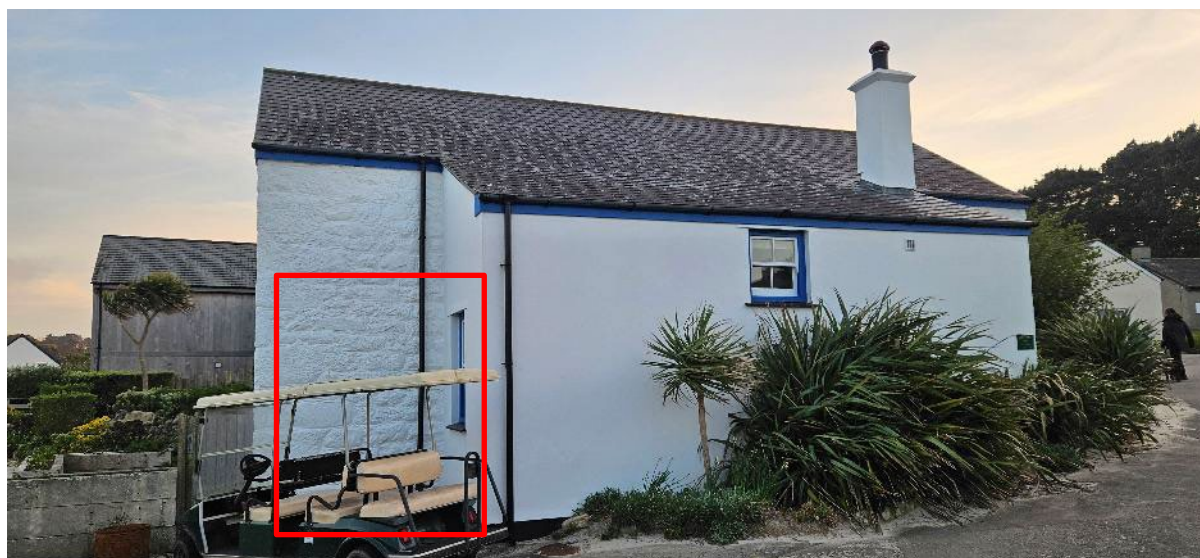
Figure 4: North elevation of Watch House; red open rectangle shows the proposed location of the single storey extension. Blue timber fascia boards above the first-floor height support a 20mm gap beneath but will not be impacted by the proposals.
