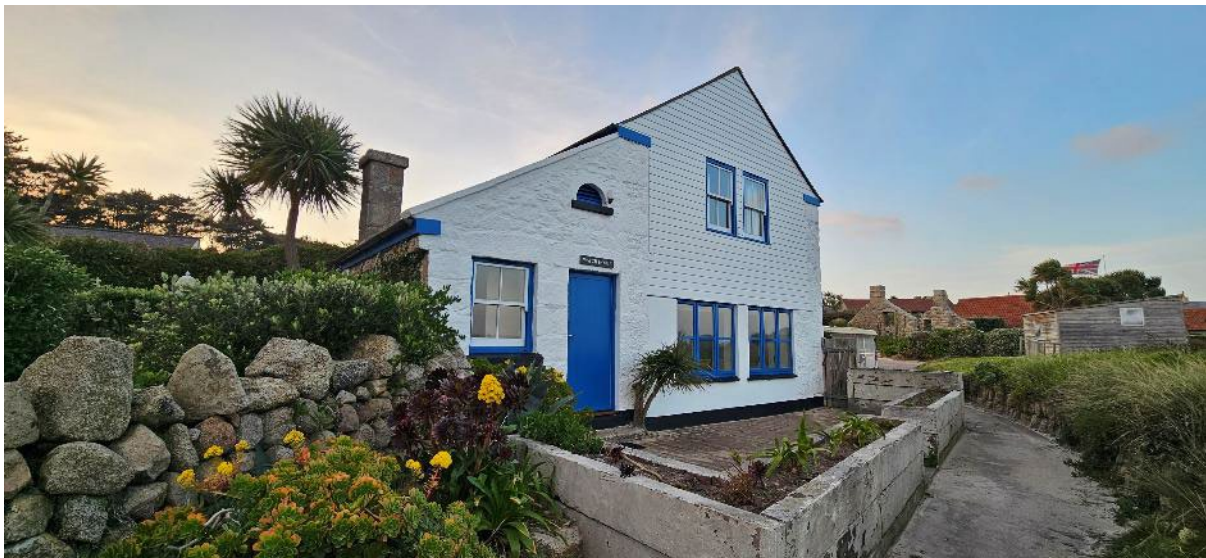
Figure 3: East elevation of Watch House showing the single storey mono-pitched projection off of the southern elevation.
