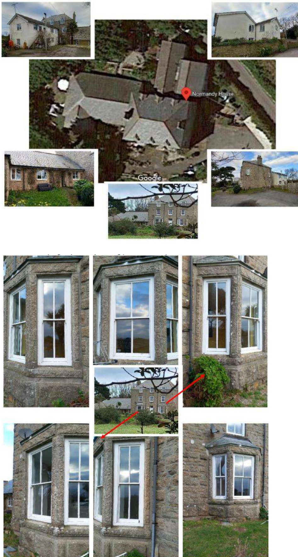
Figure 1.3: Images of Application Building from various views
