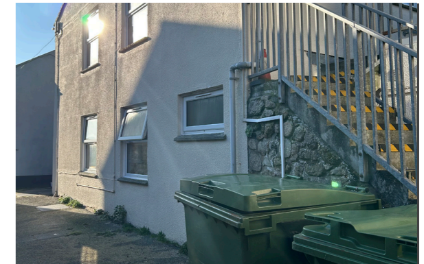
6. Side passage, yard, bins and stair
