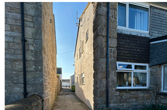
2. Passage looking south. Park House is right
