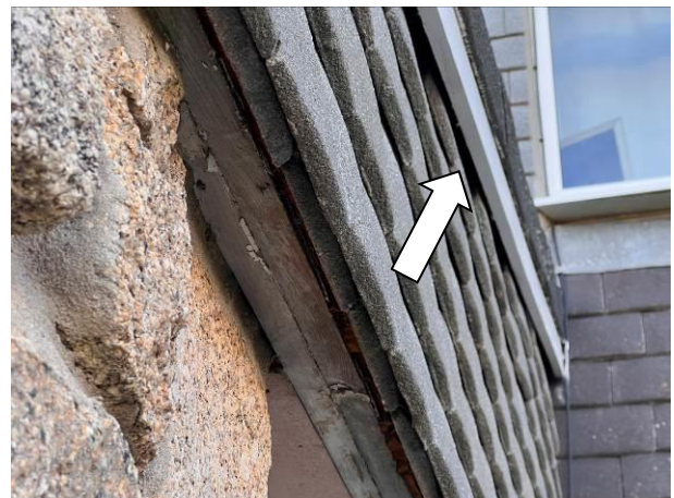
Photograph 6: Showing an example of the minor cavities present on the northern aspect where fascias overtop hanging tiles
