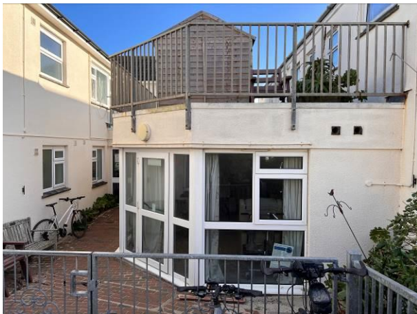
Photograph 3: Showing the flat roof component present on the southern aspect of the property.
