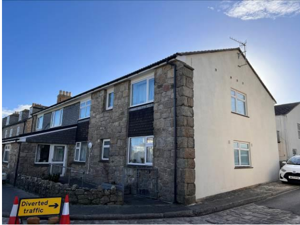
Photograph 1: Showing northern frontage and western gable of the property.
