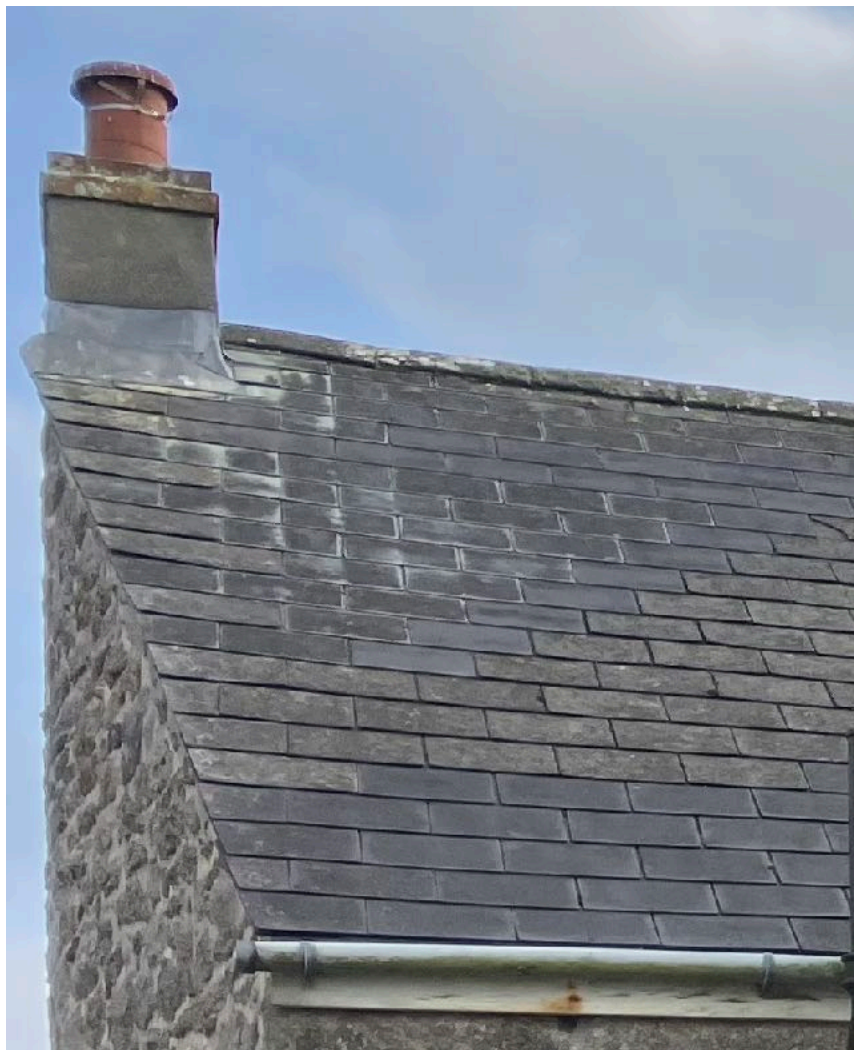
Photo image RH01 - Northerly face of East end of Rock House roof showing Asbestos cement tiles and repair tiles, with discolouration, curling, lifting, and breakage.
