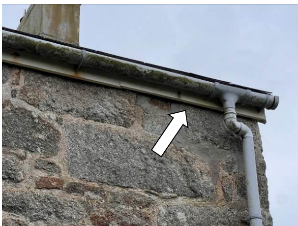
Photograph 5: Showing the eaves on the north-eastern aspect with an example of the gap behind the fascias indicated.
