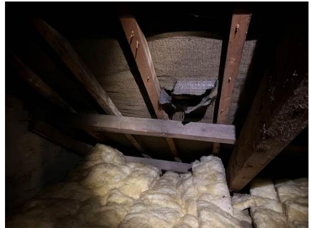
Photograph10: Showing an example of a tear in the tar paper which lies between the rafters and the battens/tiles above.
