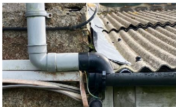
Photo Image RH03 - Westerly Face of South End of Rock Cottage showing 3 different ages and colours of rainwater goods
