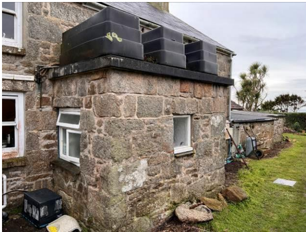
Photograph 3: Showing the water tank on the flat-roof structure.
