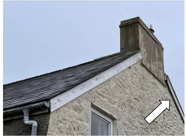
Photograph 8: Showing the south-western gable of Rock Cottage with the gaps behind the fascia indicated.
