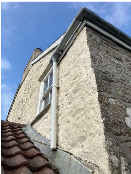
Photo image RH02 - Southern End and Easterly Face of Rock Cottage showing broken downpipes and 3 different ages and colours of rainwater goods
