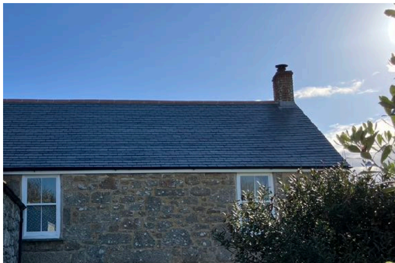
Photo Image RH05 - Dry laid and nailed Riverstone Natural Slate roof on St.Martins GV2 Listed Building - Ashdown Farmhouse - HELN 1141203
