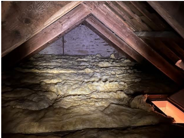
Photograph 9: Showing the interior of the loft space with insulation visible above the joists
