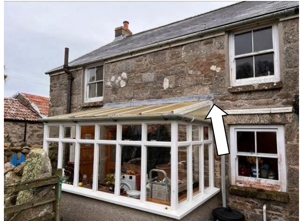
Photograph 2: Showing the north-western aspect of the property with the porch visible. The minor lifted flashing at the join is indicated.
