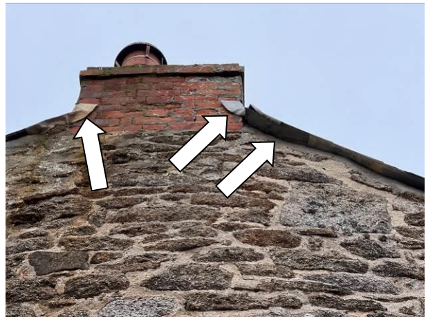
Photograph 4: Showing the north-eastern gable. Gaps beneath the chimney flashing and where pointing is missing at the verge are indicated.
