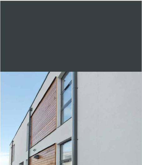
10 Aluminium pipework and hoppers to new buildings - Alumasc Squire RAL 7016
