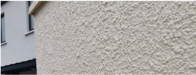
15 External Render - SIKA Parex Monorex GF Cream to match existing party wall
