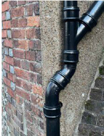
11 Cast Iron Pipework to existing building where required - J&JW Longbottom as Gutters Black
