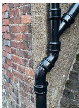
11 Cast Iron Pipework to existing building where required - J&JV Longbottom as Gutters Black
