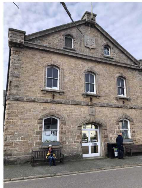
8 Timber sash and case windows
