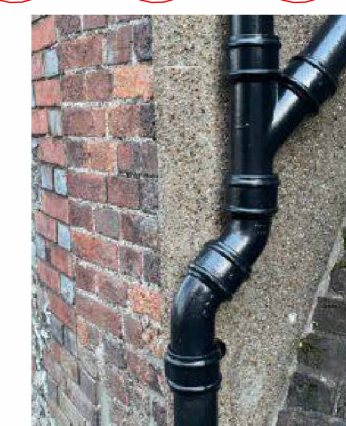
11 Cast Iron Pipework to existing building where required - J&JV Longbottom as Gutters Black
