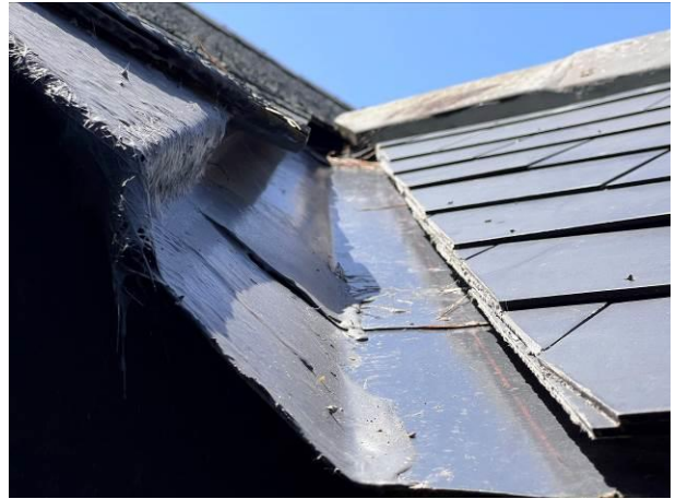
Photograph 2: Showing the well-sealed valley between the single-storey roof and the existing main pitched roof into which it is tied
