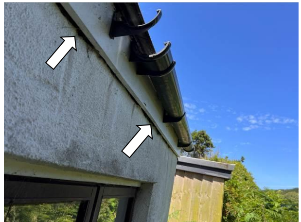
Photograph 4: Showing the gaps behind the fascia on the eastern aspect of the single-storey section
