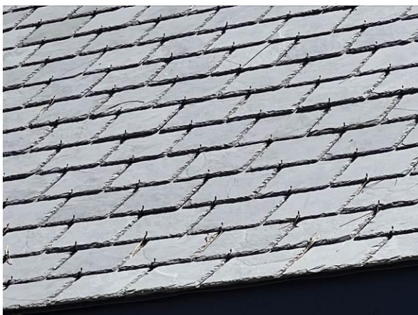
Photograph 5: Showing the tightly fitted dry-laid slate tiles of the main roof into which the new extension would be tied.
