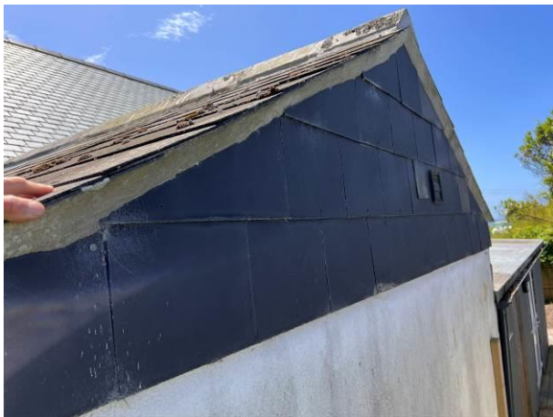
Photograph 3: Showing the hanging tiles on the upper gable of the single-storey section – these are well-sealed at the base
