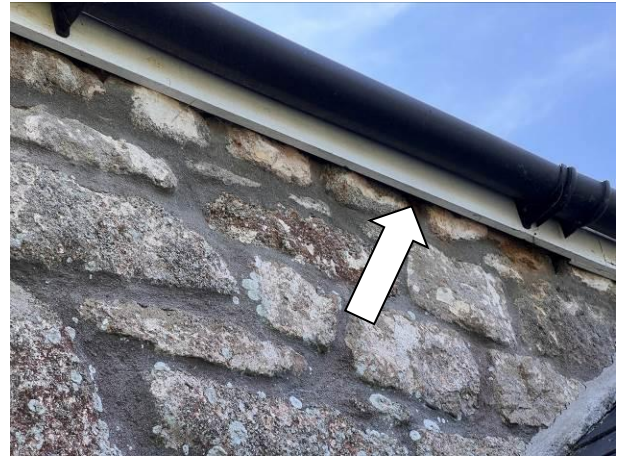
Photograph 2: Showing the fascia which runs along the eastern aspect of the two-storey cottage. This feature is present but the fly-in is obstructed on the western aspect.
