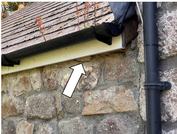
Photograph 3: Showing the fascia which runs along the eastern aspect of the single-storey extension. This feature is present but the fly-in is obstructed on the western aspect.
