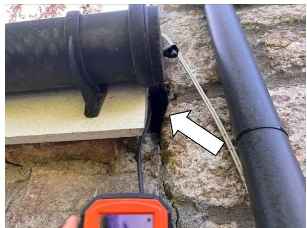
Photograph 6: Showing the gap which extends along the roofline between the single-storey extension and the two-storey cottage.
