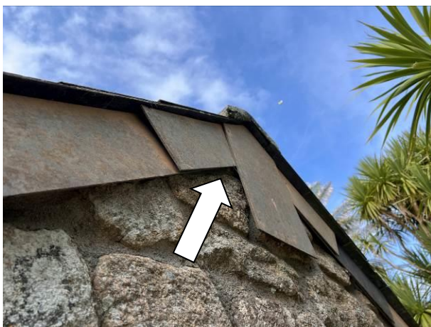
Photograph 5: Showing the drop tiles present on the southern aspect of the single-storey extension.
