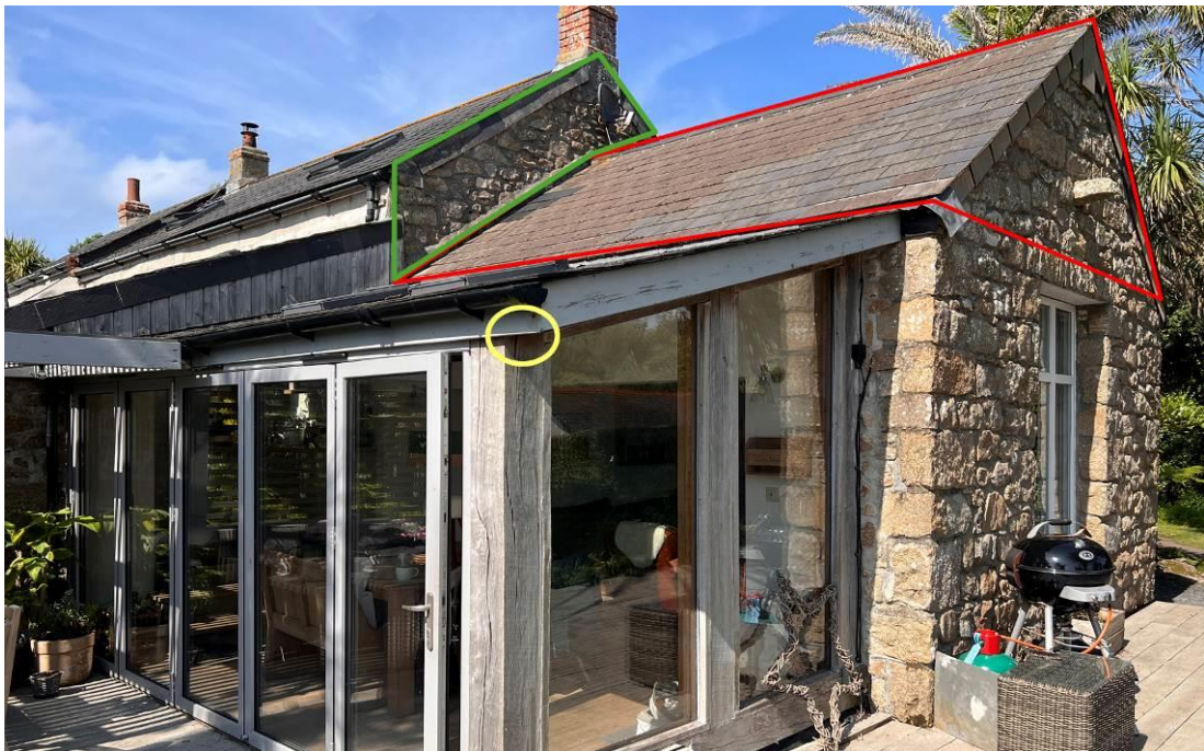
Photo 05 – Showing the structure with distinct components indicated; the single-storey extension is outlined in red - this roof would be raised to first floor level and tied in with the existing two-storey cottage outlined in green. The confirmed common pipistrelle day roost is located in the mono-pitch extension and indicated by the yellow circle.
