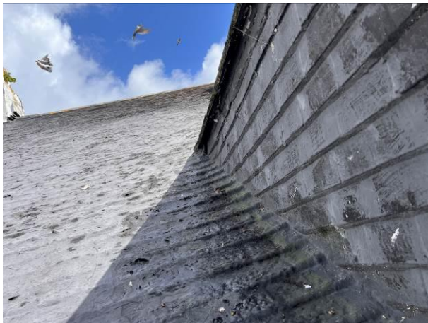
Photograph 3: Showing the bitumen painted onto the roof covering, including the hanging tiles of the dormer.
