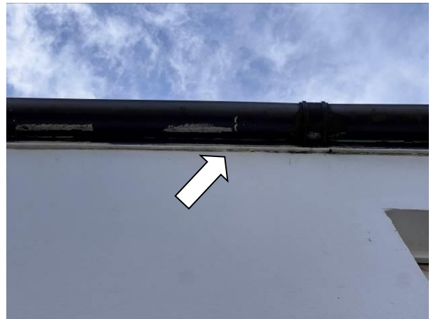
Photograph 4: Showing the tightly fitted fascia on the eastern aspect of the main house.
