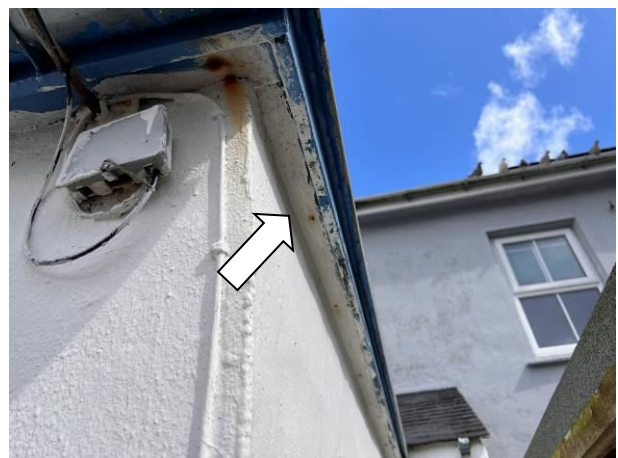
Photograph 6: Showing the tightly fitted fascia on the single-storey extension.
