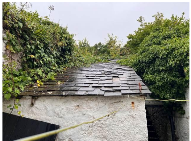
Photograph 6: Showing Outbuilding B with the natural slate tiled roof. The gaps between slates close to the eaves practice can be seen.
