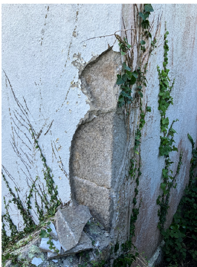
Figure 1: Showing dressed granite beneath render
