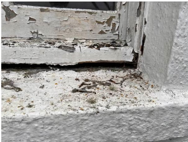
Photograph 3: Showing an example of the rot present in some window frames which does not yet offer roosting opportunities for bats but may develop in time.
