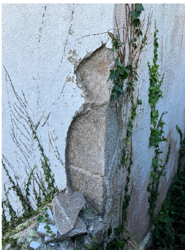
Figure 1: Showing dressed granite beneath render
