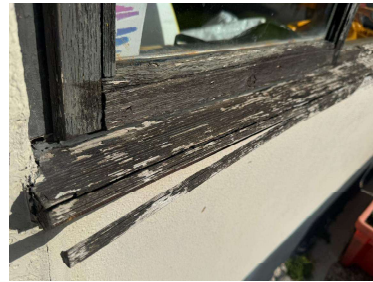
Photos showing rot and decay Of existing windows
