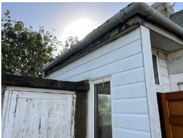
Photograph 5: Showing the flat-roof extension with uPVC cladding.
