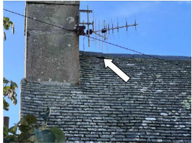
Photograph 2: Showing the roof structure – this is largely well-sealed with no gaps noted; however occasional minor gaps are noted including the gap in the ridge highlighted.
