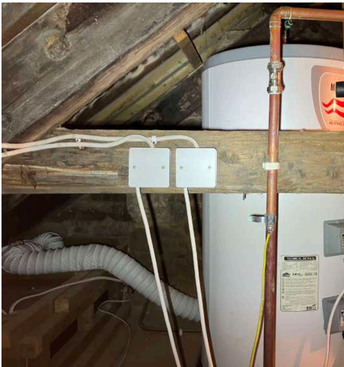
Figs. 39-40: Existing flexible ventilation duct within loft, serving existing shower room and terminating through roof. To be reused.
