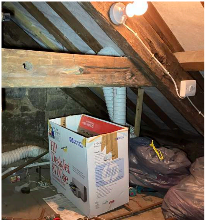
Figs. 39-40: Existing flexible ventilation duct within loft, serving existing shower room and terminating through roof. To be reused.
