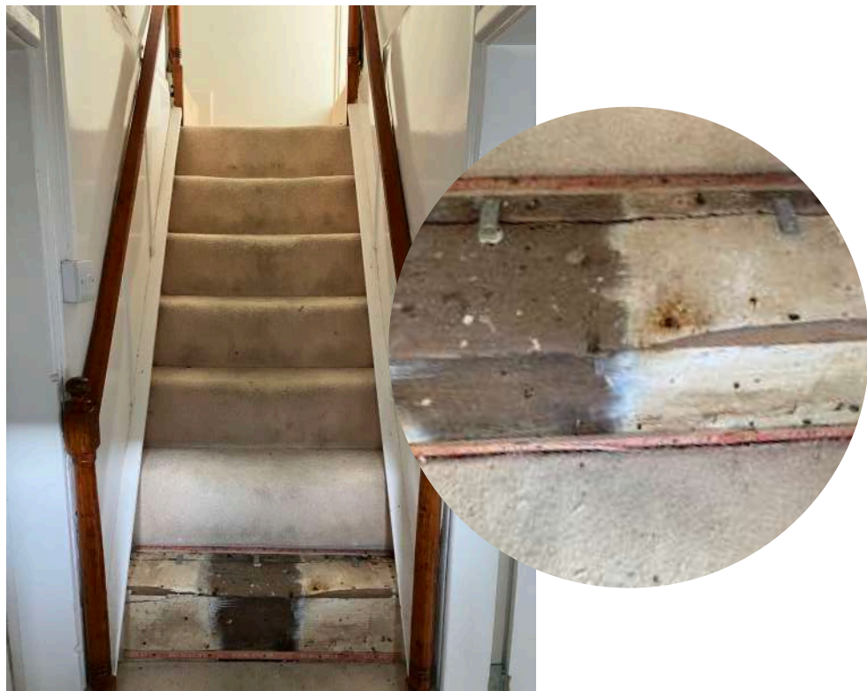
Fig. 28: Stairs, with insert to demonstrate poor state of repair of stair
