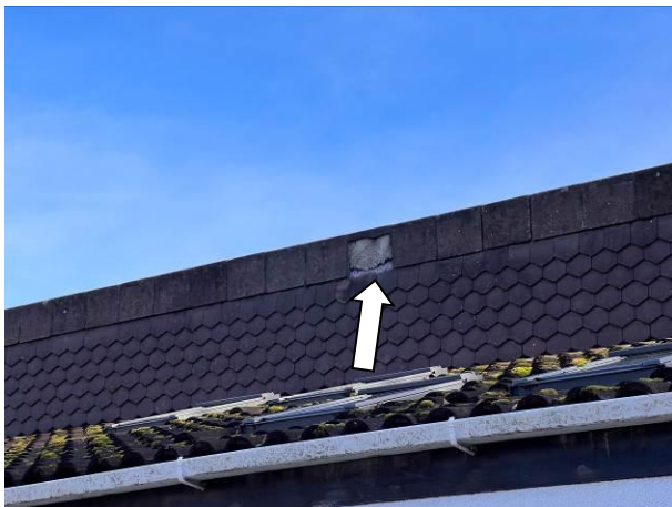
Photograph 3: Showing an example of the damaged drop tiles on the western ridge of the main structure.
