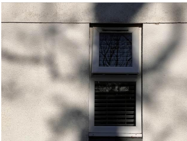
Photograph 5: Showing an example of the uPVC windows whose frames are well-fitted within the apertures.
