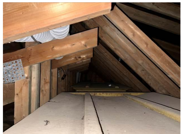
Photograph 6: Showing the interior of the loft space – this image includes the cover of the water tank below, whereas the majority of the loft space has insulation between the joists.
