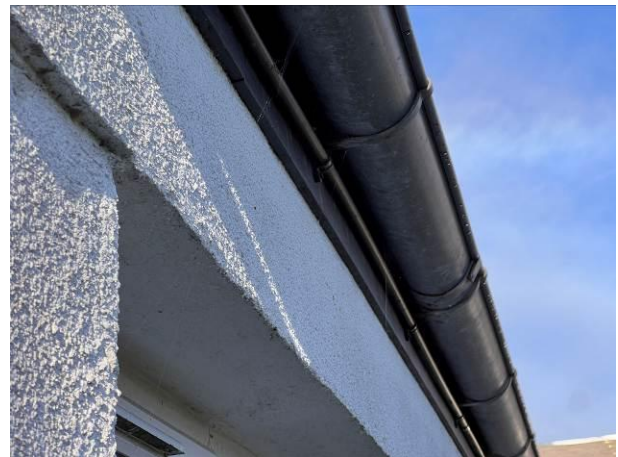
Photograph 4: Showing an example of the tightly-fitted fascia along the eastern aspect of the building.
